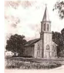
Historic St. Paul Church, Bayou Goula, Louisiana
